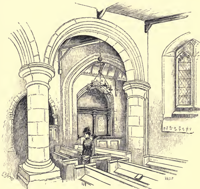
INTERIOR, SPARSHOLT CHURCH.
